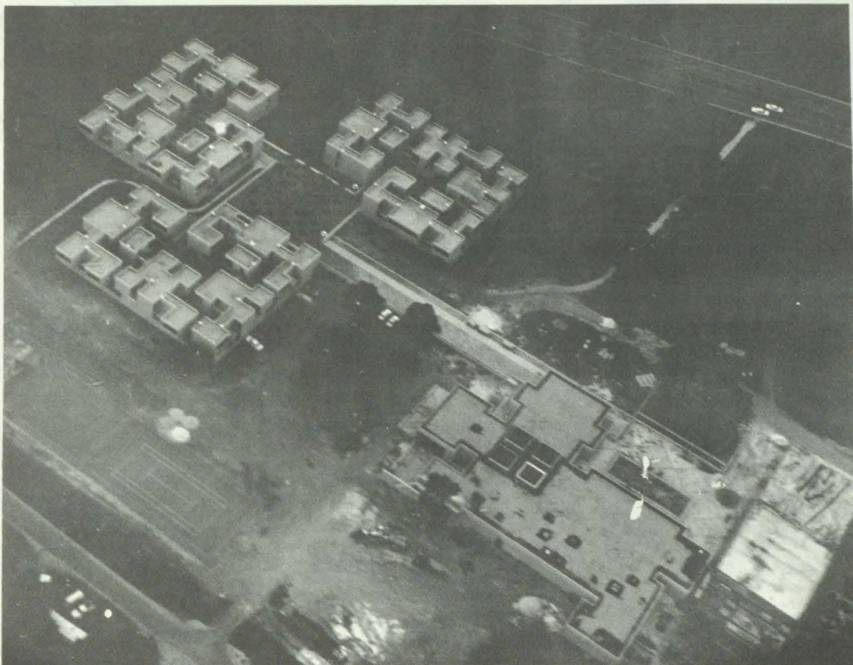
Hamilton Court construction is proceeding very slowly, as the general contractor continues to have difficulties with area labor organizations. The outer construction is virtually completed, however, as this aerial photo taken at dusk shows. The three dormitory courts are toward the upper left, and Hamilton Court lies on the lower right.
