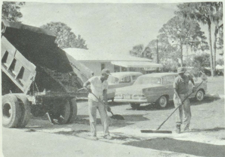
WEST CAMPUS ROADS were re-surfaced this week. The major work was completed Thursday, with minor repairs still continuing.
