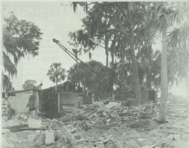
Some of the old army barracks were torn down this week on the east campus as construction work continues to "move along well" on the Hamilton Court project. Planning Officer Ralph Styles expressed confidence this week the latest target date--Feb. 15--will be met.
